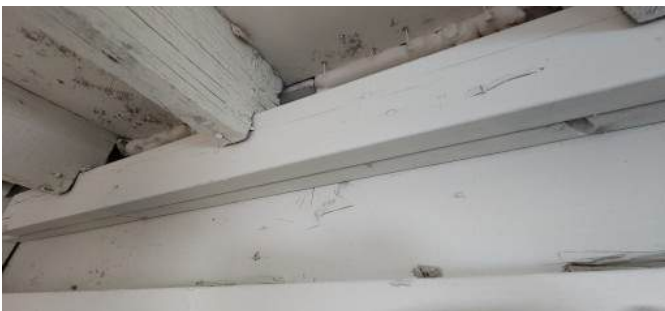
Joists are resting on a 2"x4" nailed to a 2"x4". (gym area)
