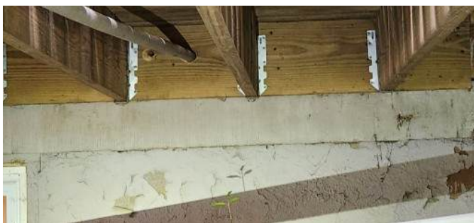
Lag bolts are the preferred method of attachment.
