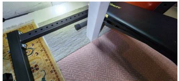
Wood support is sitting on the floor. (gym area)
