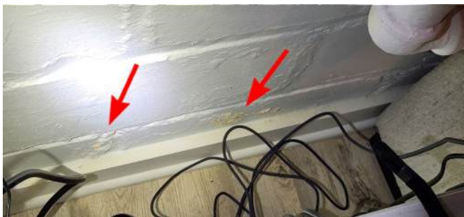
Efflorescence.
