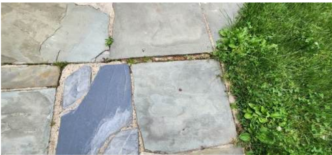
Missing/cracked mortar.
