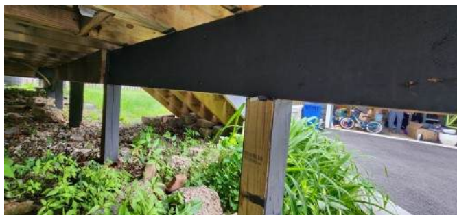
Posts in contact with the ground.
