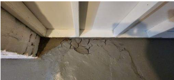
Cracked floor.
