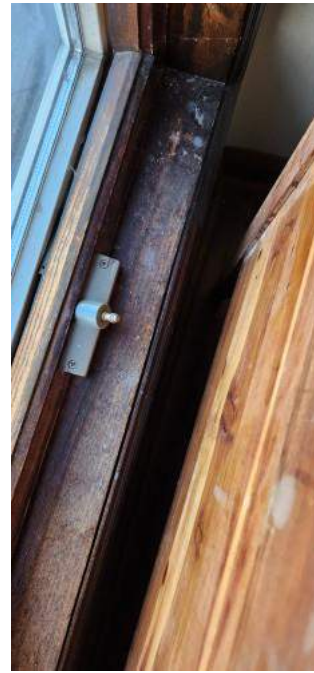
Missing casement crank.
