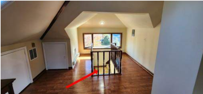
Loose guardrail. Balusters too far apart.
