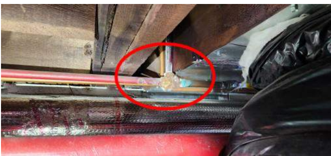
Pipe has been leaking here. (right of washer/dryer)
