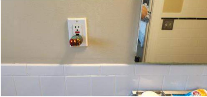
Reversed polarity.
