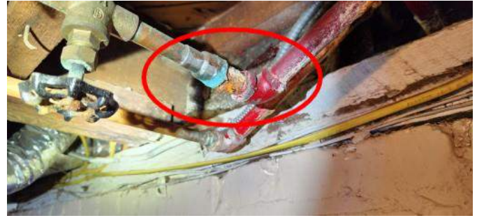
Indications of a leak. (back left of basement)
