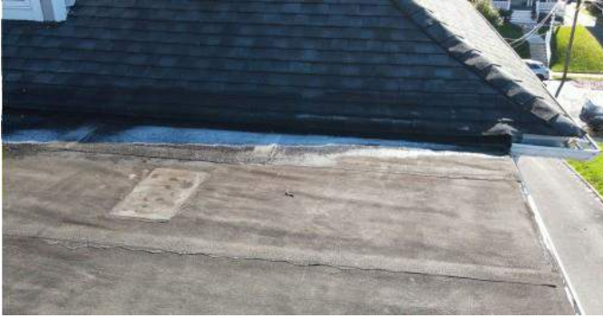
Flat roof is cracking.
