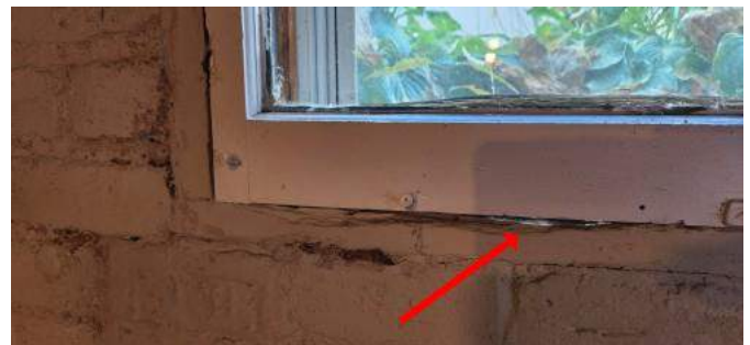
Nailed shut. Weather-stripping needed to seal drafts.
