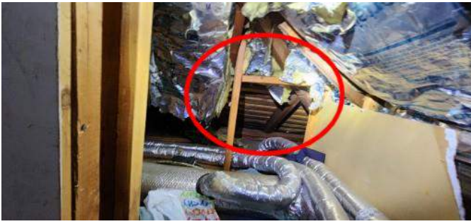
Missing insulation.
