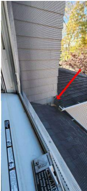
Missing wood shingle. (rear of house)
