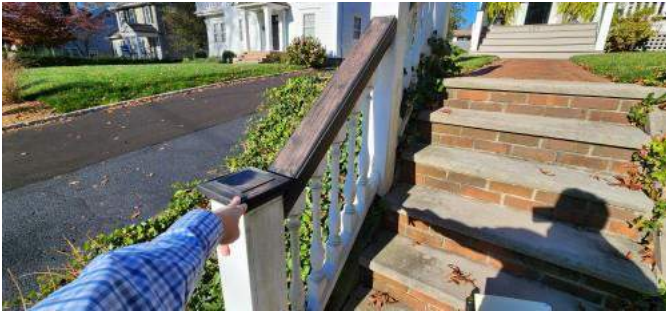
Loose handrail.
