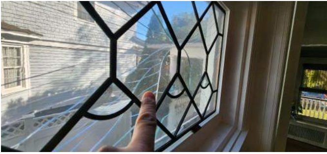
Exterior window at the stained glass was broken.
