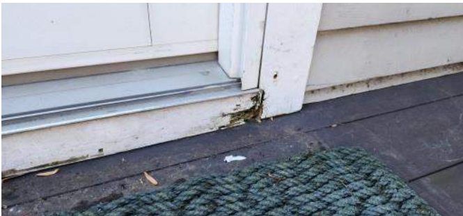
Board under the door sill was rotten.
