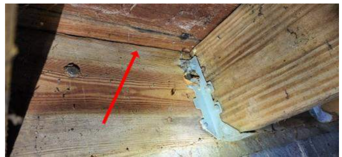
No flashing visible.
