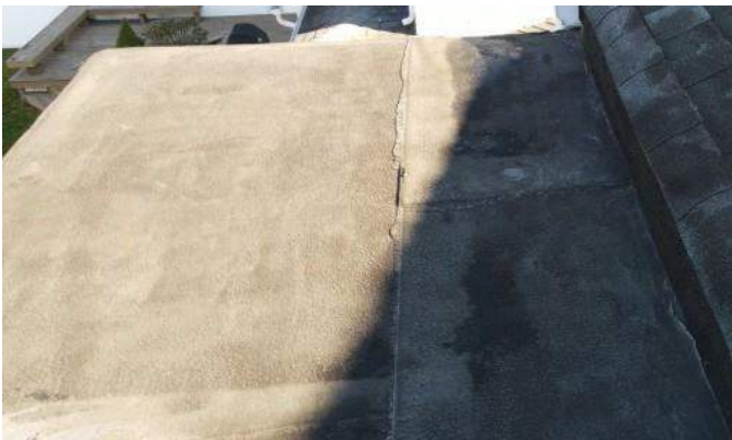
Flat roof is cracking and likely at the end of its life.
