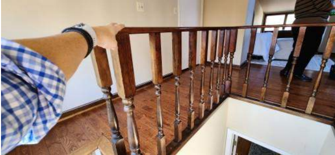
Loose guardrail.
