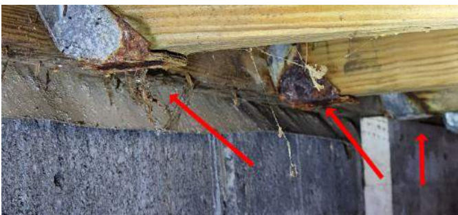
Rusted joist hangers.
