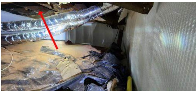
Missing insulation.
