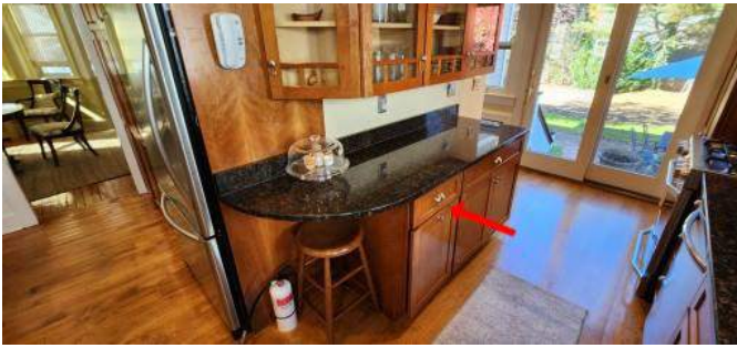
Drawer pull missing screw.
