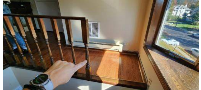
Missing guardrail.
