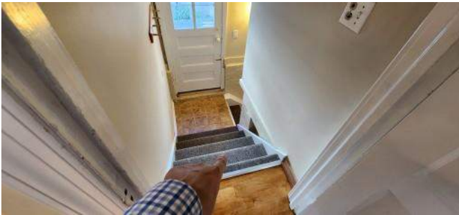
No handrail at basement stairs.
