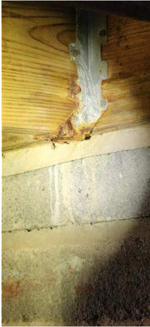
Rusted joist hanger.
