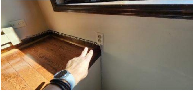
Ungrounded outlet at the top of the stairs.
