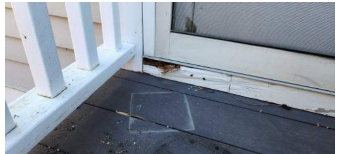
Board under the door sill was rotten.
