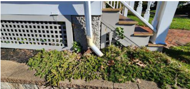
Downspout empties into underground drain.
