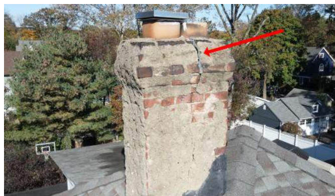
Major cracks and deterioration.
